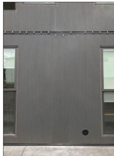
- Slip the new panel into place and face fasten panel - Putty the screws and use touch-up paint to cover
