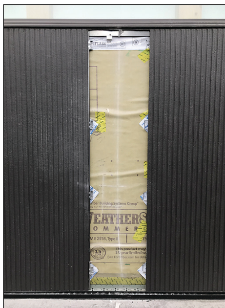
- Break and remove damaged panel
