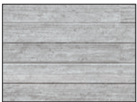
Board Formed Concrete
