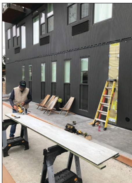
- Cut lap joint off new panel and set spacer blocks
